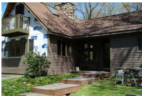
Front view of the home.
